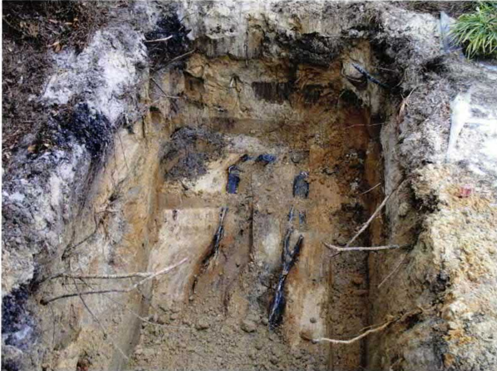
Picture 2: Excavation in progress.
